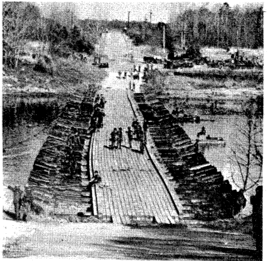
The busy crossing at Engineer Landing as constructed by members of Co D, 43rd Engr Bn the 586th Engr Co (Float Bridge).
