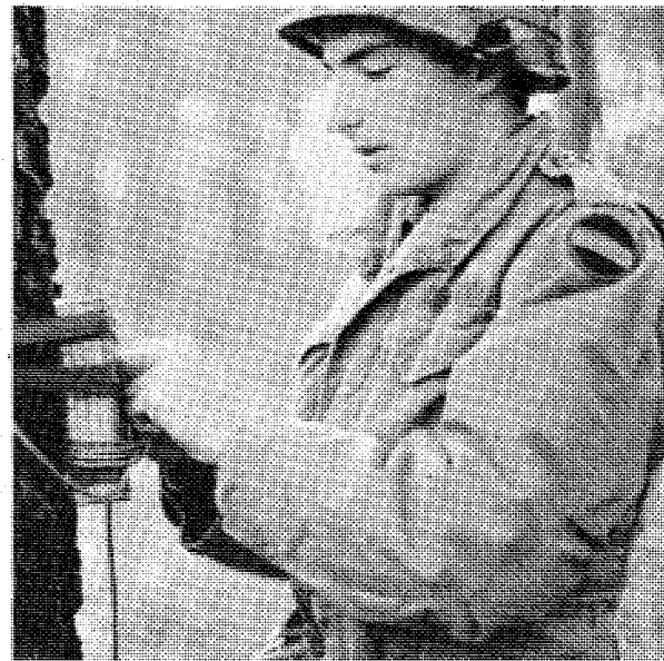
Pvt. 2 Daniel Caprio ties detonating cord to the TNT to secure the charge to the tree.
