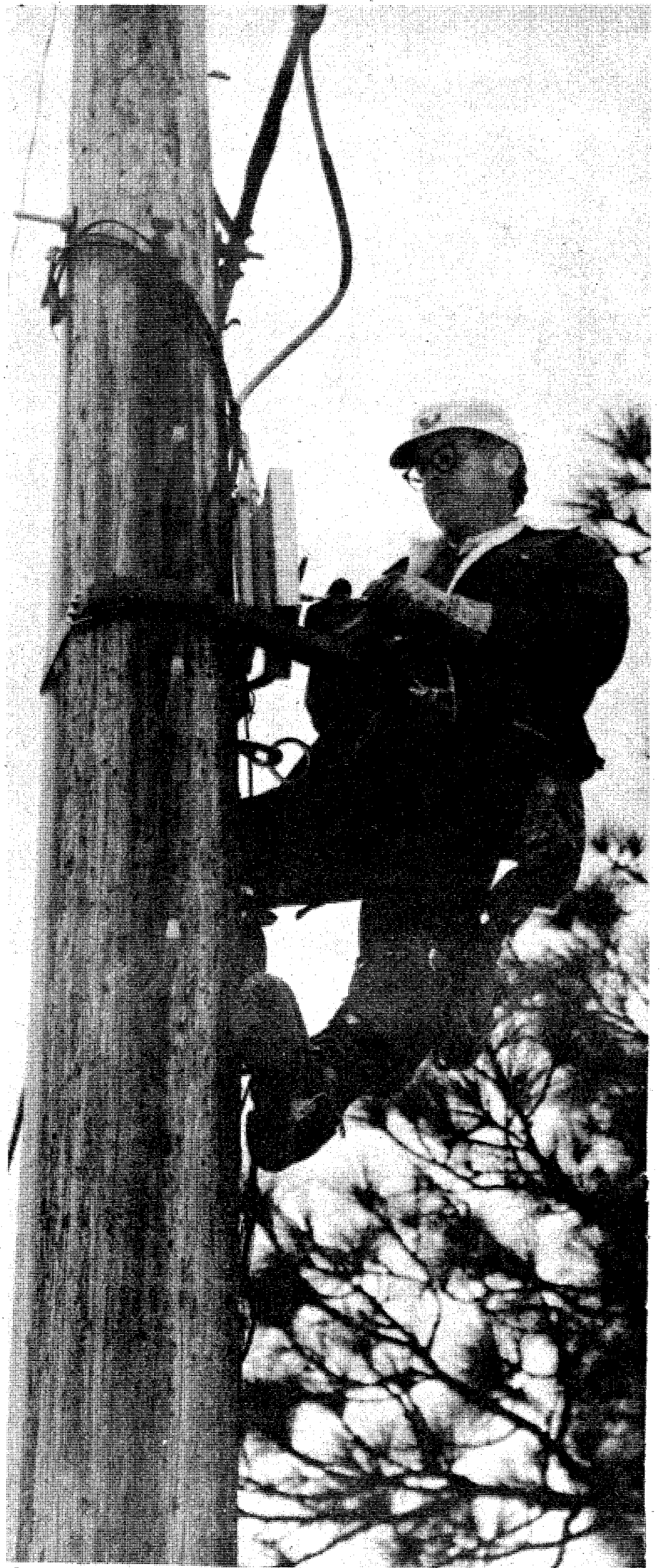
An Outside Plant cable repairman checks out a terminal on a multi-pair cable.
